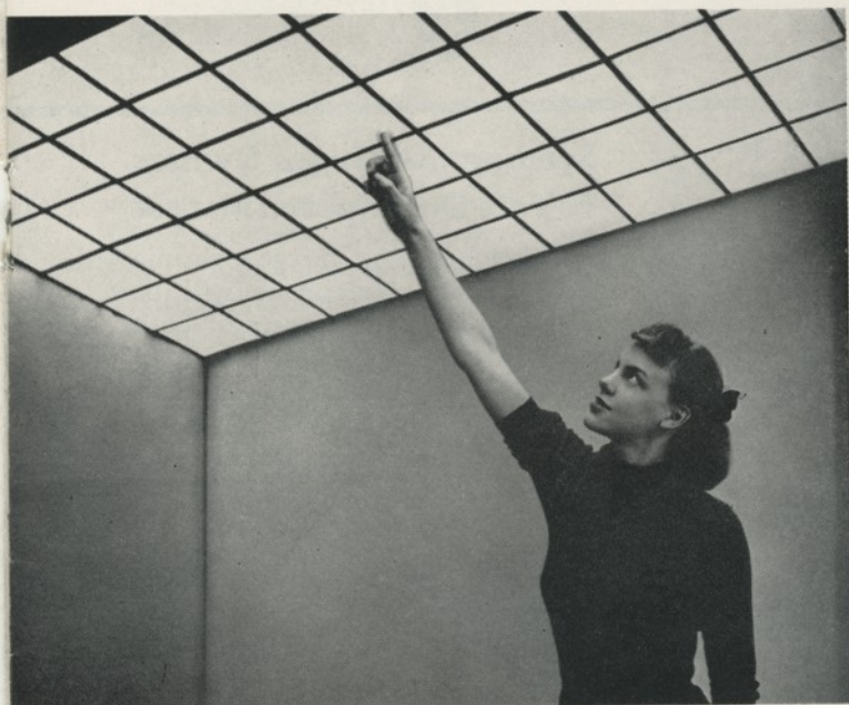
This ceiling is lighted by many "Panelescent" lamps. Through research, the company's laboratories have developed phosphors which increase lamp brightness using same power.
